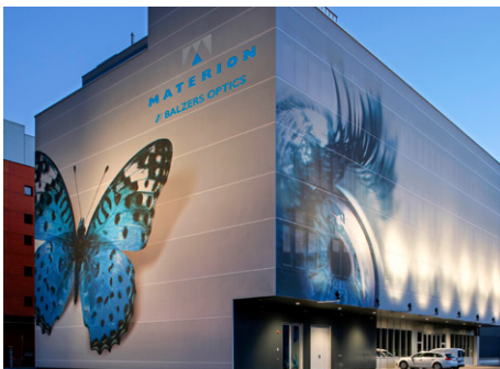
Production Balzers/Principality of Liechtenstein
